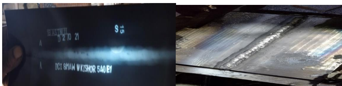
Figure 7. (Radiography testing) rt and (visual inspection) of 9 welded plate
