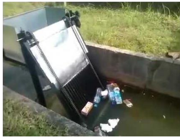
Figure 3. Automatic drainage cleaner.
