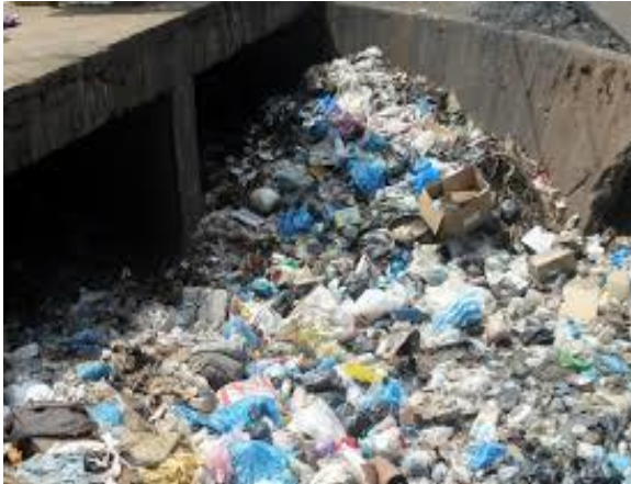
Figure 2. Coagulation of drainage with plastic waste.
