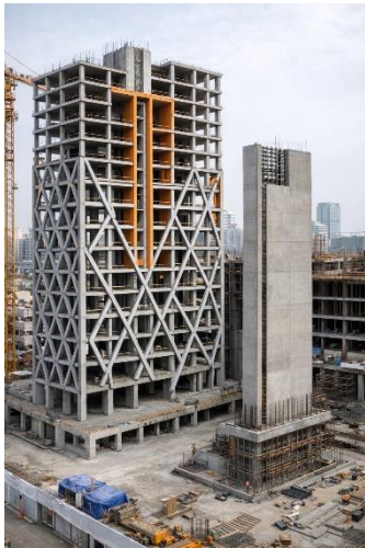
Figure 2. RC Shear wall.
