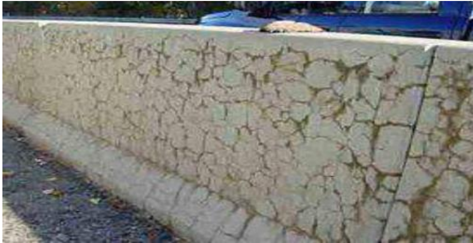
Figure 4. Typical Effect of Alkali-Aggregate Reaction.
