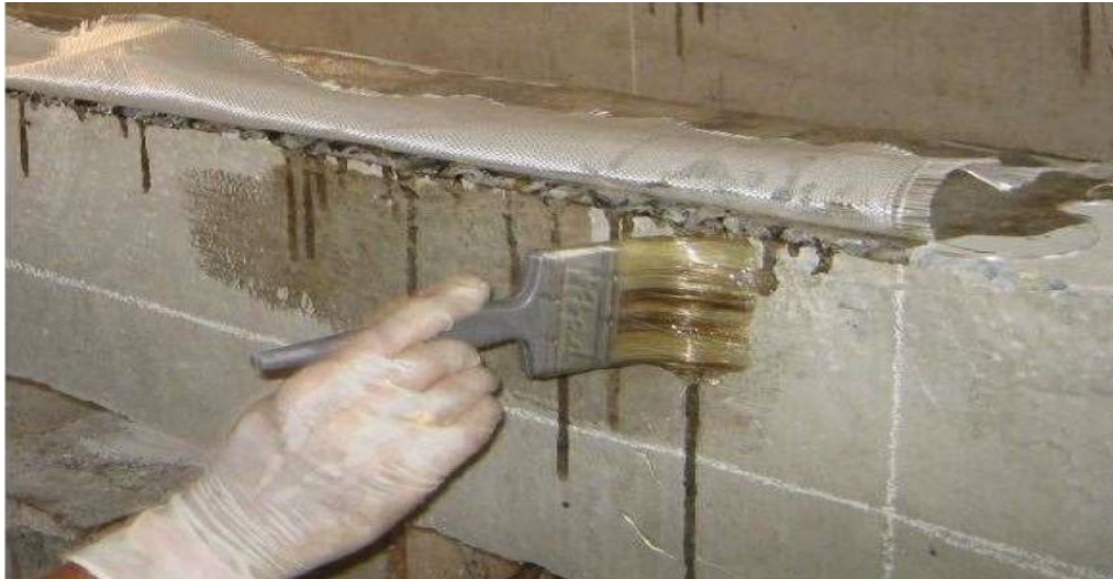
Figure 12. Application of Primer Coat or Coupling Agent.
