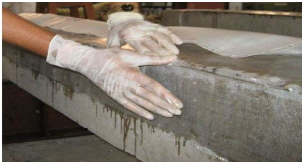
Figure 13. Application and Fixing of GFRP.
