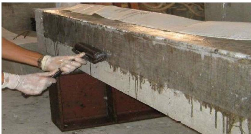
Figure 14. Removal of Entrapped Air.
