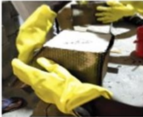
Figure 4. Wrapping of FRP
