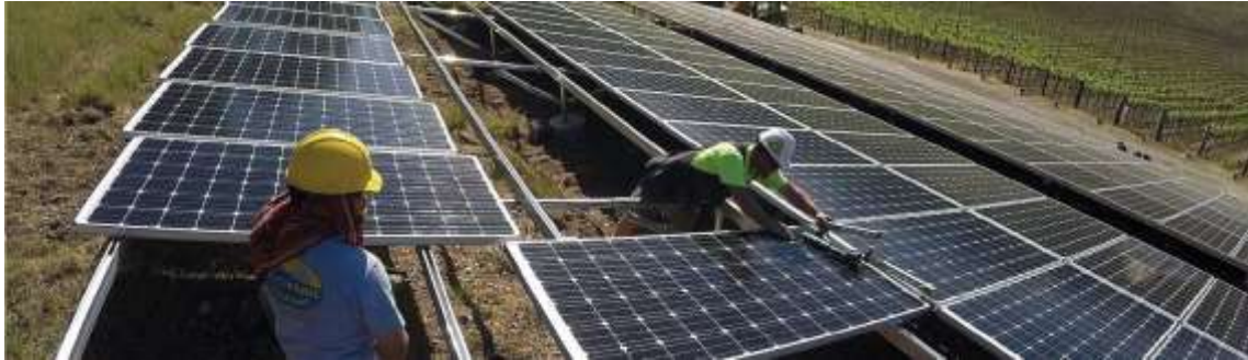
Figure 1. Manual cleaning of solar panel module.
