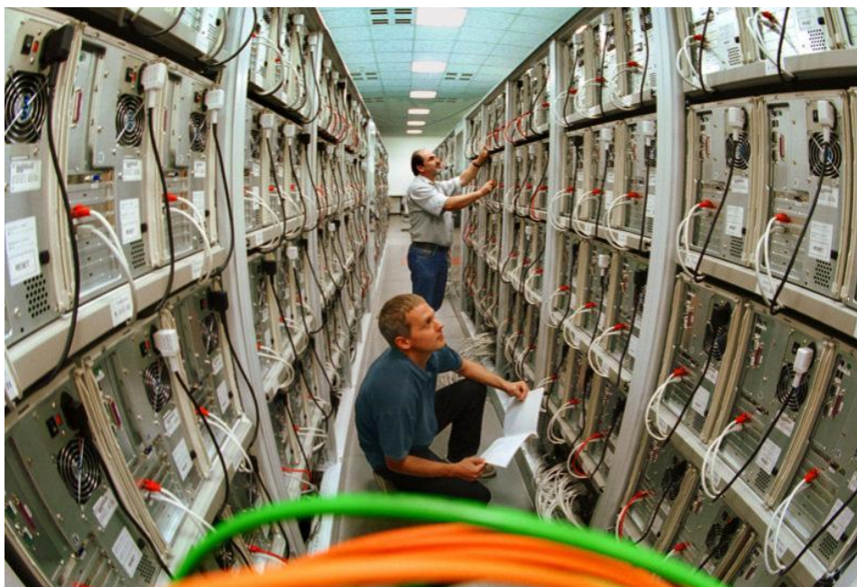
Figure 2. Technicians working on a cluster consisting of several servers.
