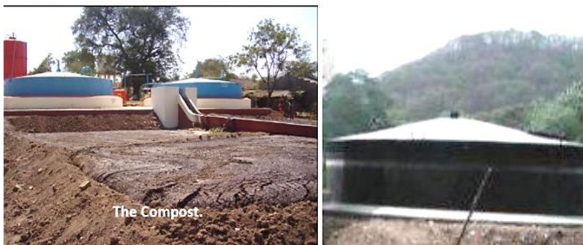
Figure 32. Bio gas plant.
