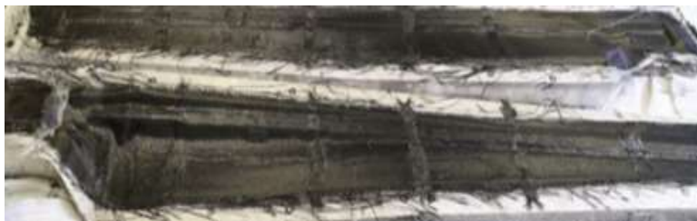
Figure 5. Placement of epoxy resin and jute fiber layups.
