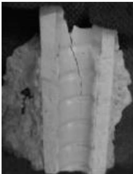
Figure 3. Cover splitting on concrete cracking.
