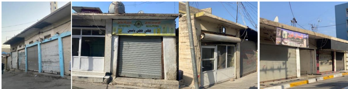
Figure 10. Roofing: Reinforced concrete roofs which belongs to era after 1950s.
