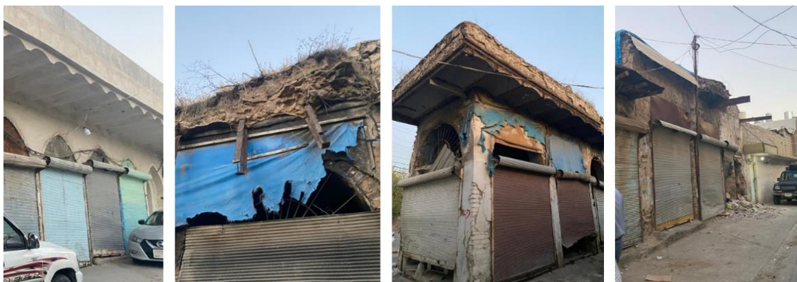
Figure 8. Roofing: Steel section supported roofs belongs to the era pre 1950s.
