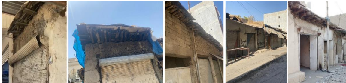
Figure 9. Roofing: Timber tree trunks, it was the local material build by local workers.
