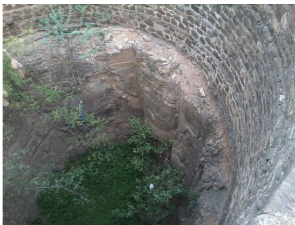
Figure 13. Section showing compact massive basalt at Gawalewadi.
