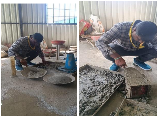
Figure 2. Concrete mixing for slump cone and cube.
