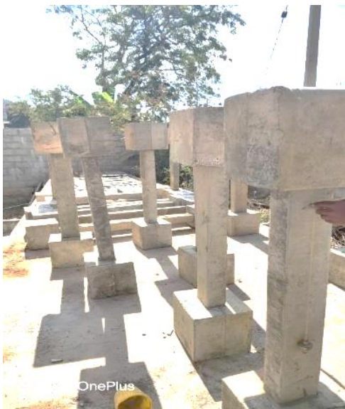
Figure 6. Cast columns
