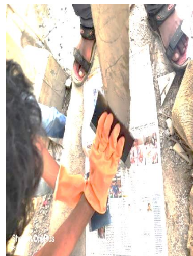
Figure 13. Applying bond material for precast
