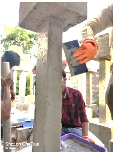
Figure 12. Applying the bond material for column
