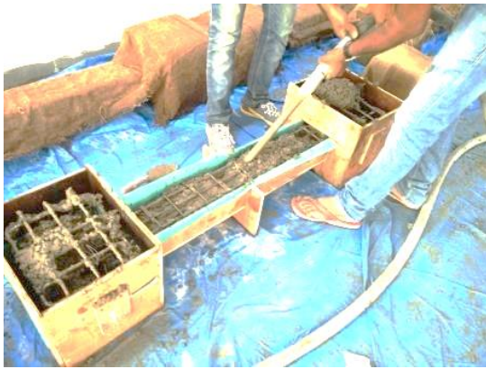
Figure 5. Casting of columns
