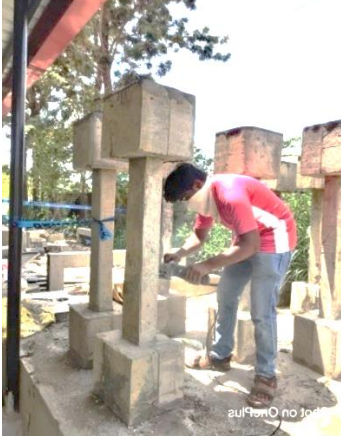
Figure 11. Grinding of columns
