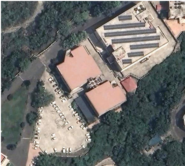
Figure 2. Vastu, school of architecture and planning.
