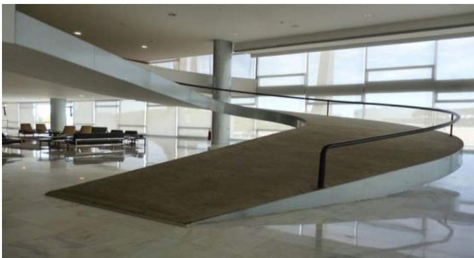
Figure 14. Ramps for easily accessible.
