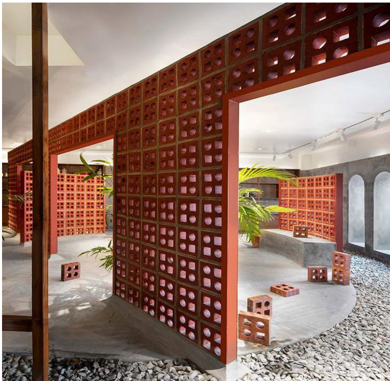
Figure 34. Sustainable material partition wall.
