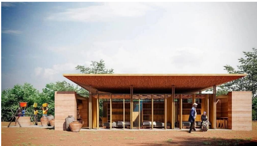
Figure 1. Exterior view of the Tanzanian family house showing rammed-earth walls, bamboo screens, and an elevated cooling roof.
