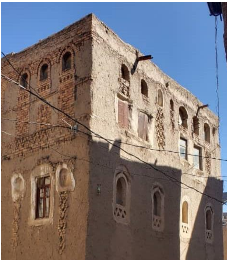
Figure 7. House built from brick and mud.
