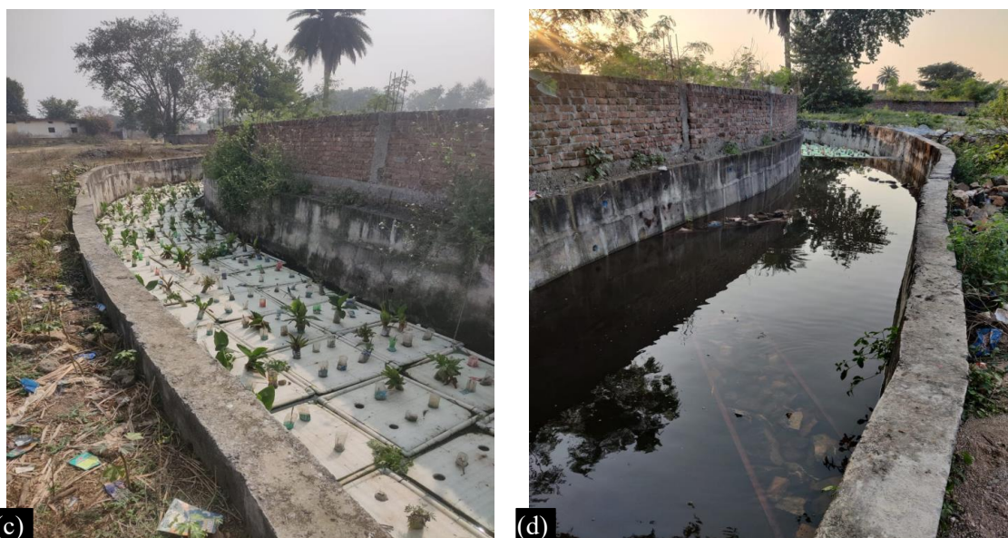
Figure 1. (a–d) Plants Implementation on Drain Water for Phytoremedial Treatment.
