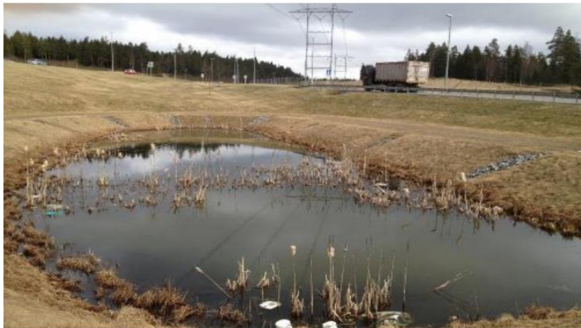
Figure 3. A norwegian sedimentation pond with a forebay and a main Pond.(Photo: Sondre Meland, Source:Lensa Jotte Et Al. 2017) [16]
