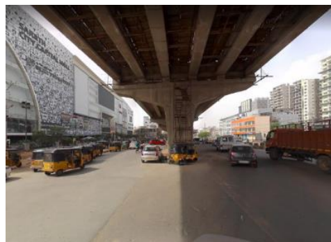
Figure 18. (b) Under the Kothaguda Flyover, To the left is the Sharath City Capital Mall (Source-Google maps).
