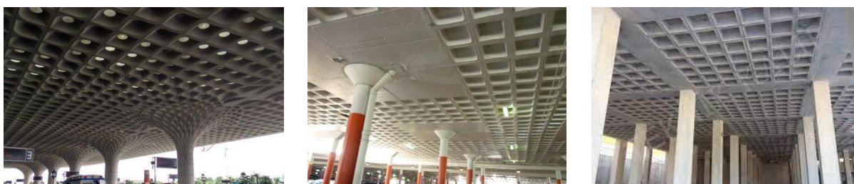
Figure 1. Waffle slabs.
