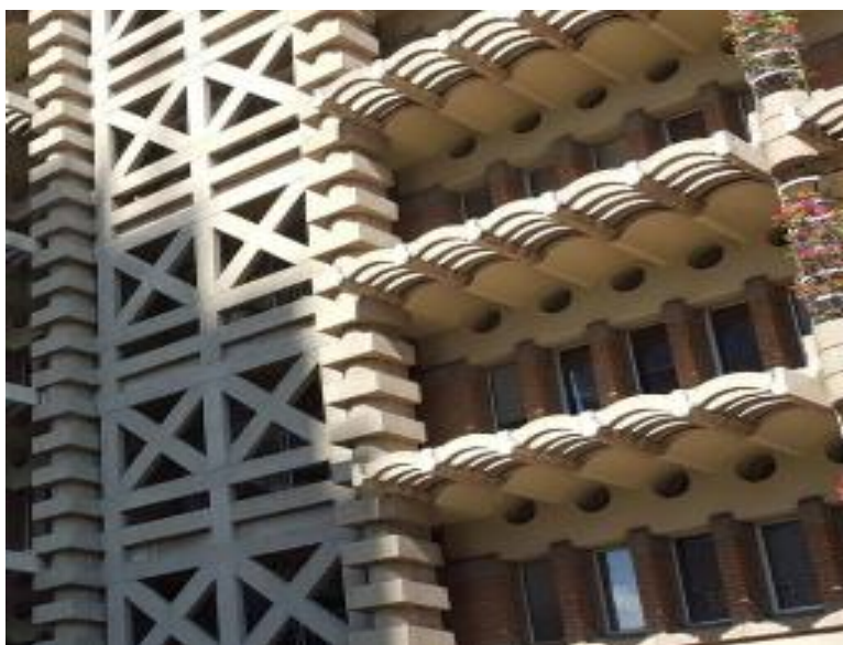
Figure 11. Concrete prickly bodies that act as a sunshade. Source: Stefan Novakovic, How Architects Are Getting Innovative and Addressing the Climate Crisis , www.threemagazine.com [13].
