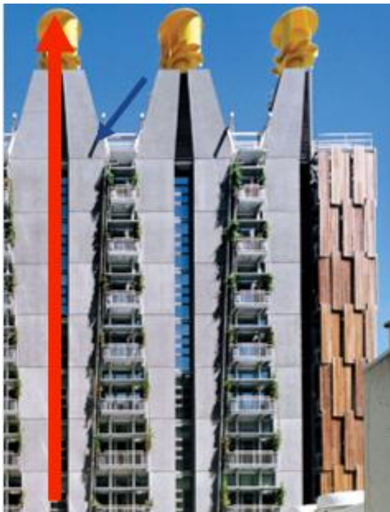
Figure 6. Chimney with wind turbines at the top for air circulation. Source: Nancy Yen-Wen Cheng. 2017 [7].
