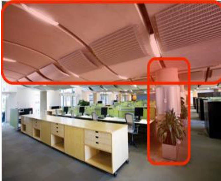
Figure 5. Curved ceiling and columns with high thermal mass. Source: Nancy Yen-Wen Cheng. 2017 [7].
