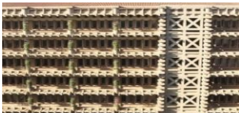
Figure 9. Concrete prickly bodies with high thermal mass.
