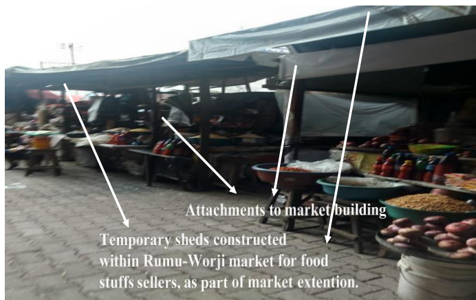
Figure 7. Image showing the use of zinc as an attachment space in Rumu-Woji market.
