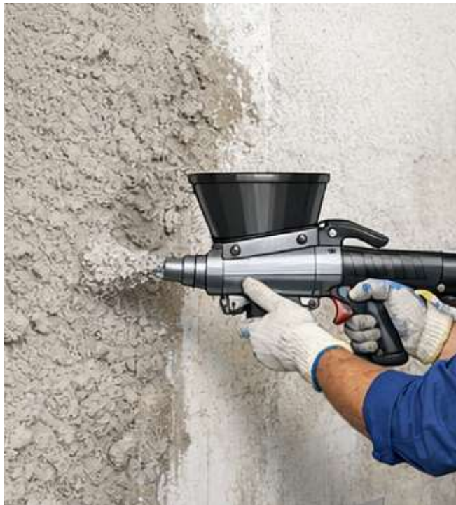
Figure 9. Intended operator interaction with the polymer–metal hybrid spray assembly during wall plastering.
