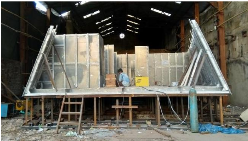
Figure 11. Fabrication of Aluminium super structure.
