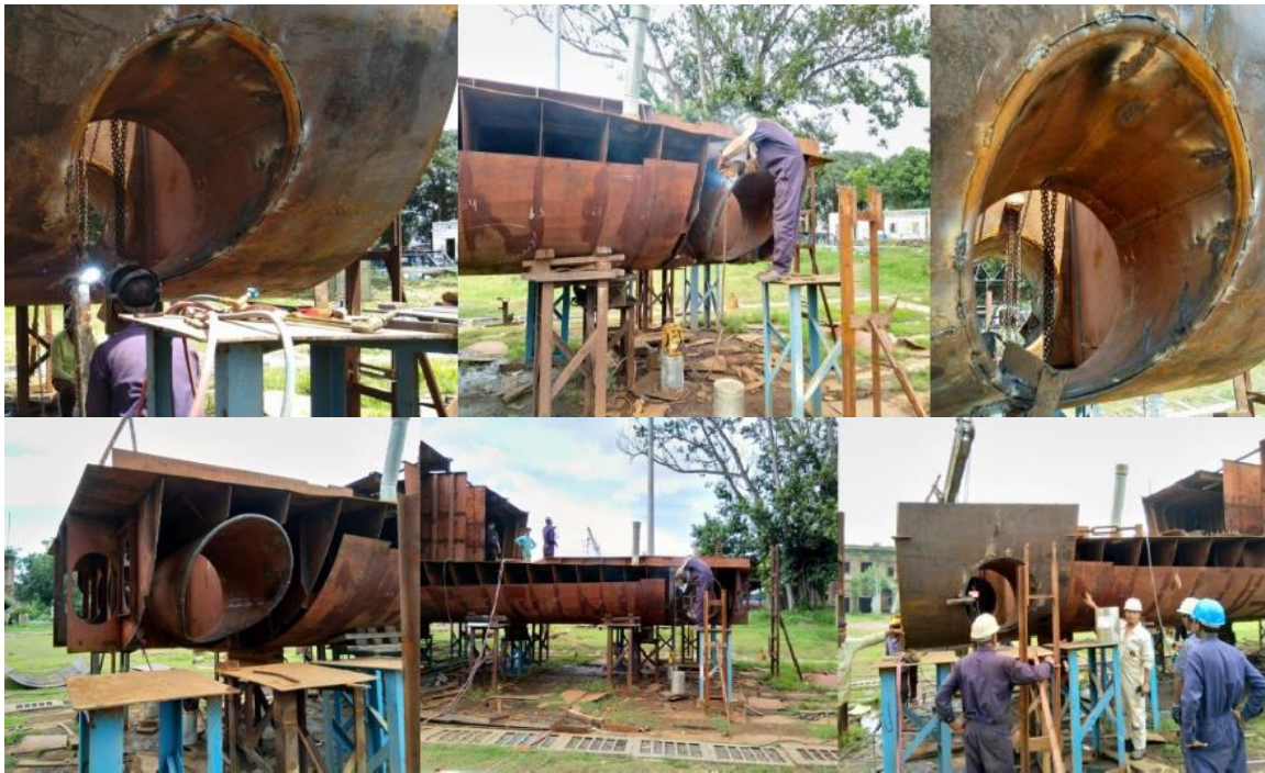
Figure 7. Block Fabrication work in progress at yard.
