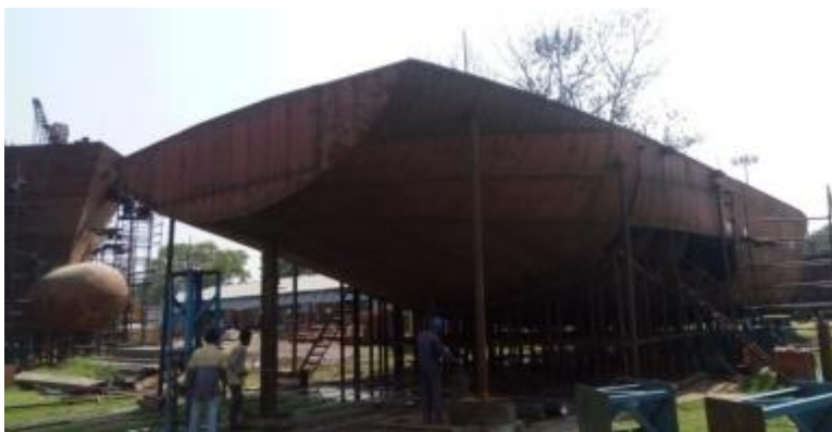
Figure 5. Ship block fabrication at shipyard.
