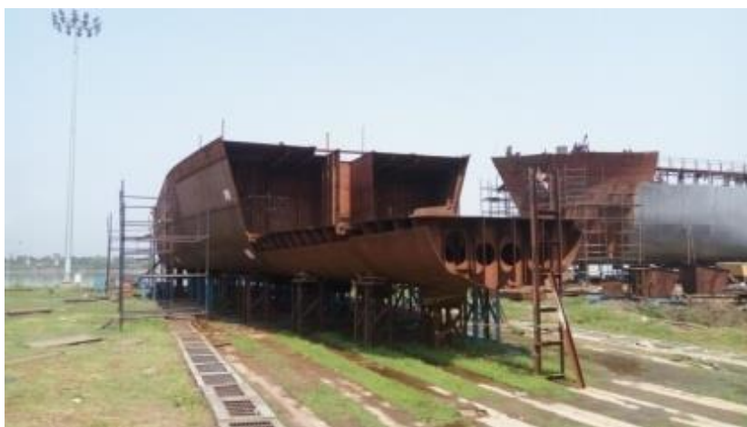
Figure 4. The ship hull construction at the shipyard.
