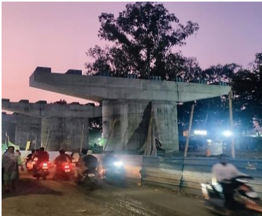
Figure 3. Reti Mandi Flyover overbridge construction.
