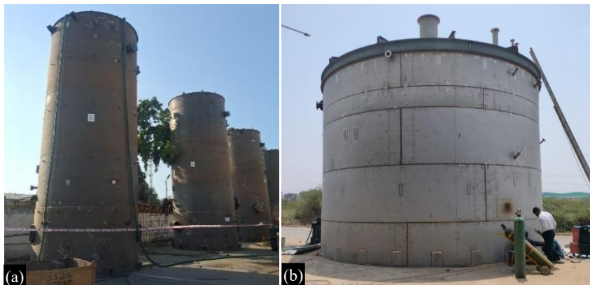
Figure 13. Hydro test—water filling test.
