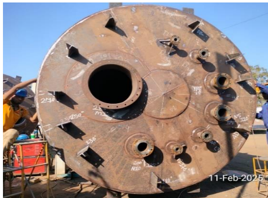
Figure 4. Storage tank roof.
