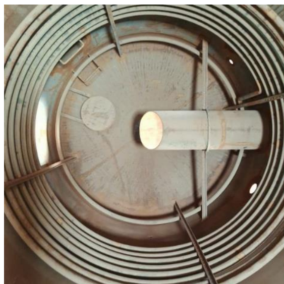
Figure 14. Hydrotesting of the coil inside the storage tank.
