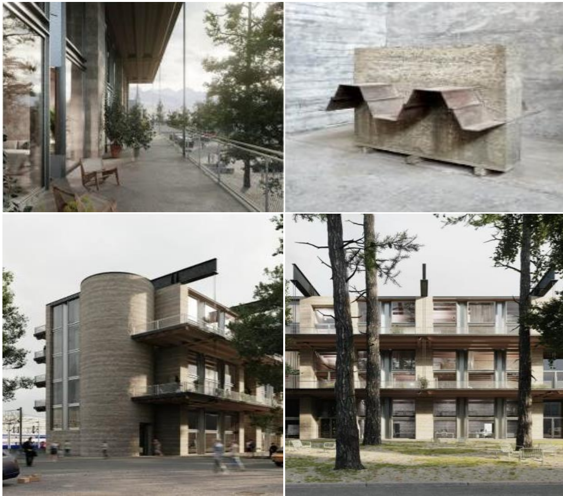
Figure 17. Steel building structure in different view.
