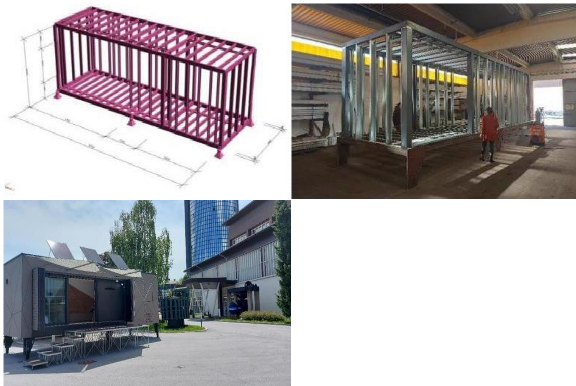
Figure 19. Construction of steel house.
