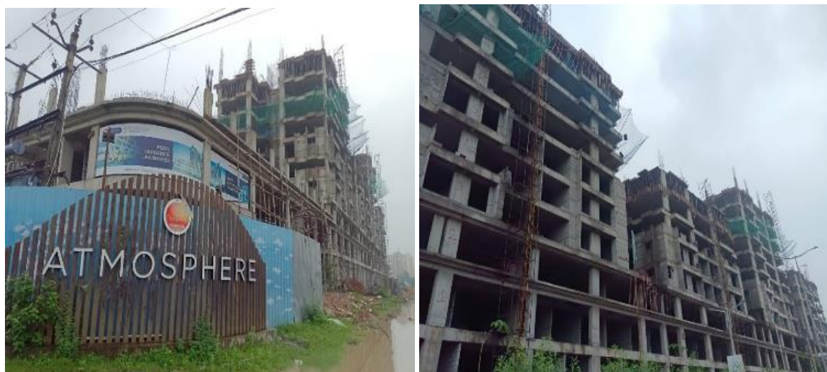
Figure 11. On-site construction photos.
