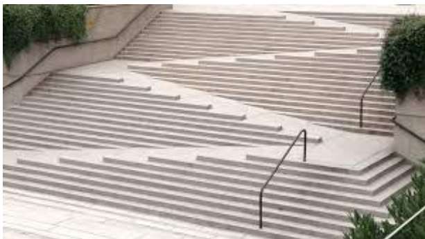
Figure 10. Accessible staircase for all.
