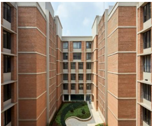
Figure 27. Courtyard in the center of the hospital.
