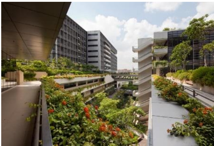
Figure 18. Green courtyard can be seen from the hospital premises above the floors.
