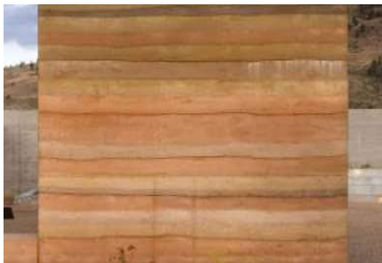
Figure 3. Rammed earth wall.
