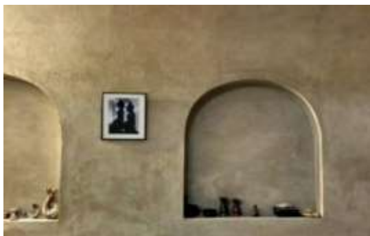
Figure 5. Clay and lime plaster used for interior walls
