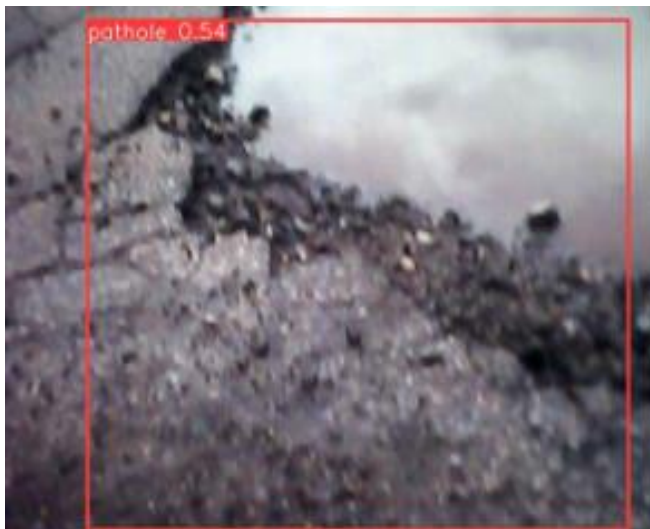
Figure 5. Pothole detected by YOLOv5 (Pathole-0.54).
