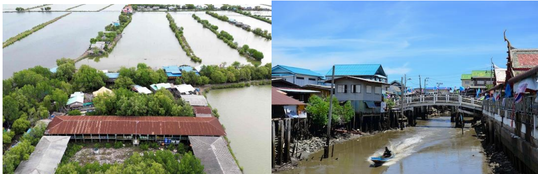
Figure 2. Floating house project in Ban Khun Samut Chin.
